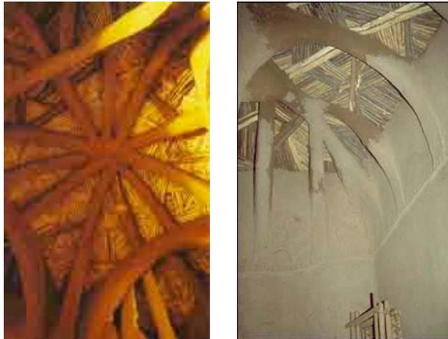
Figure 6: Yaama dome interior with square base and hemispherical top; and latticework beneath adobe plaster (from <http://www.islamicity.com/Culture/Mosques/Africa/TMp192b.htm> and [http://archnet.org/library/images/thumbnails.jsp?location\\_id=1914](http://archnet.org/library/images/thumbnails.jsp?location_id=1914)).
